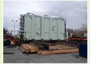
The crew constructed a temporary pad to support and store the transformer until the substation was ready to integrate it. They then utilized a jack and slide system to move the unit directly from the railcar to the pad. After setting the transformer, the crew unloaded several trucks of transformer accessories into the yard for storage as well. The entire job was completed safely and on time.
