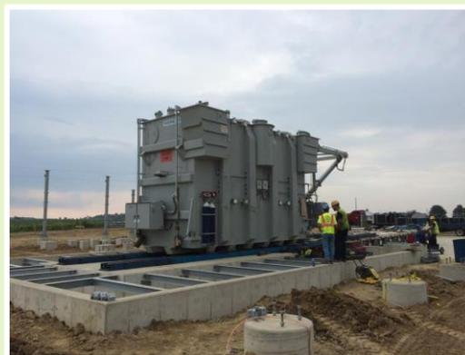
The dual lane trailer hauled the unit to the site in Lynn, IN, but was too large to directly access the final pad. HLI therefore employed the gantry system to transload the unit onto a 6 line goldhofer which was small and agile enough to haul the unit to a position adjacent to the pad in the proper orientation. The crew then used a jack and slide system to load the transformer from the trailer to the final pad where it awaited final installation.
