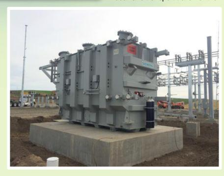
With the transformer secured, the trailer began the slow and deliberate haul to the final destination substation. Once alongside the concrete pad constructed to receive the unit, the riggers again utilized the jack and slide system to load it from the trailer onto the foundation. There the new transformer awaited final assembly and assimilation into the substation. The project was completed safely and on time.
