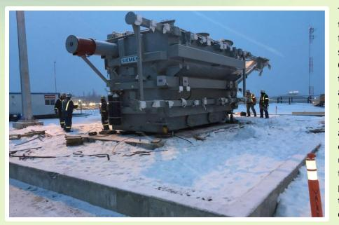
The crew carefully hauled the transformer over the snowflecked roads to the receiving substation in Dawson Creek, AB. Once on site, they maneuvered the trailer to a position alongside the pad to facilitate the offload, but the limited space prevented them from achieving the proper orientation of the transformer. HLI again utilized a jack and slide system to offload the transformer to the pad where they used a turntable to spin the transformer to the correct alignment.
