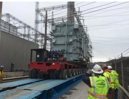
In April, HLI coordinated the replacement of a power transformer at a site in Stratton, OH. The crew started the four day job with the removal of the old unit. They jacked the timeworn transformer up to the trailer elevation and slid it onto the self-propelled modular trailer with a hydraulic jack and slide system. Next, the team carefully maneuvered the trailer through the crowded substation to a crib pile in a designated area and offloaded the unit for storage there.
