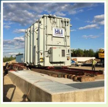
HLI railed this 243,380lb unit from Laredo, TX to a rail siding in Milford, ME. After arriving at the rail siding, the transformer had to be offloaded from its heavy duty rail car to an over the road transport system to be delivered to the substation. The best choice for offloading this heavy transformer from the rail car and loading the large transporter was using a jack and slide system.
