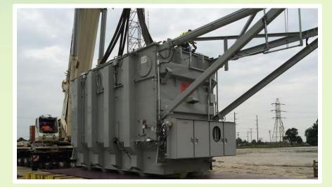
Now loaded, the transformer made its way to the substation. Upon arrival, HLI chose a crane to complete the off load. The riggers picked the unit off the transport trailer and placed it safely on its temporary pad, ready to be installed at a later date. The job was completed safely, on time, and within budget.
