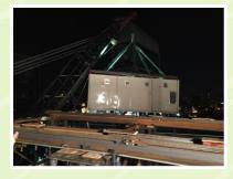
HLI incorporated the use of a barge crane for this complex job due to access restrictions and the cranes maneuverability, to lift 2 boilers onto the hospitals roof. Prior to the lift, HLI and associates had to design a support and runway to skate the boilers from the barge crane landing location, a lift frame to accommodate both boiler units, and verify the integrity of the roof structure to support the slide operations.
