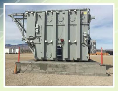
HLI railed this 265,145 lb. unit from EI Paso, TX to a rail siding in Rosamond, CA. At the rail spur, HLI employed the jack and slide system to slide the transformer off the railcar and place it onto a specialized girder transport trailer for the subsequent haul to the site.
