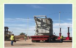
HLI railed this 257,530 lb. unit from Eagle Pass, TX to a rail siding in Dodge City, KS. After arriving at the rail siding, the transformer had to be offloaded from its heavy-duty railcar to an over the road transport system to be delivered to the substation. HLI chose a Gantry system for offloading this heavy transformer. The Gantry had to be assembled and disassembled a number of times during the various stages of this move.
