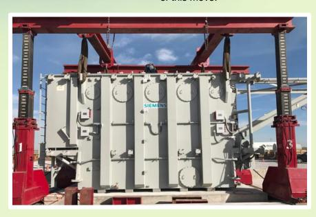
After inspection of the transformer, it was lifted off the rail car, and placed on the transporter to haul to its destination. After a safe arrival at the substation location, it was removed from the transporter using the Gantry system. Once the transformer travelled over the pads retaining wall, it was set on slide rails and slid over to its final installation pad.
